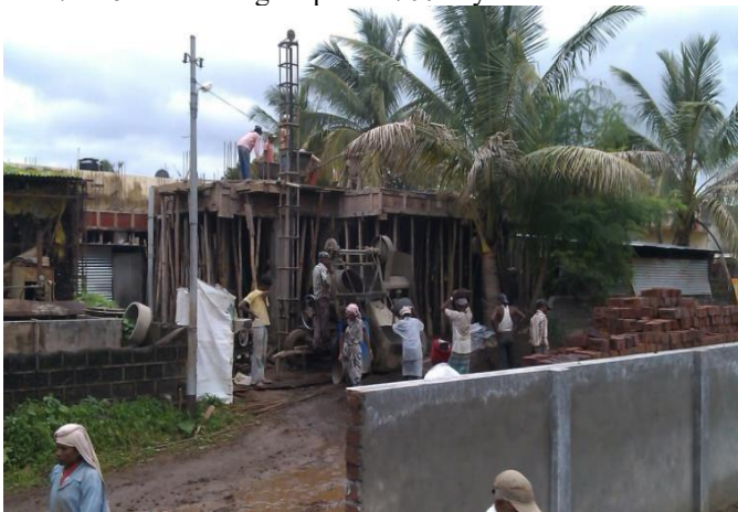
(Fig 3) On-Site Mixing in One-bag mixer
