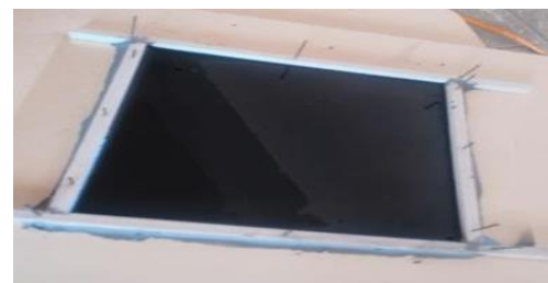
Fig 6. Shows fabrication of layer 5
