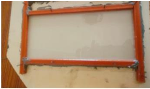
Fig 2. Shows fabrication of layer 1
