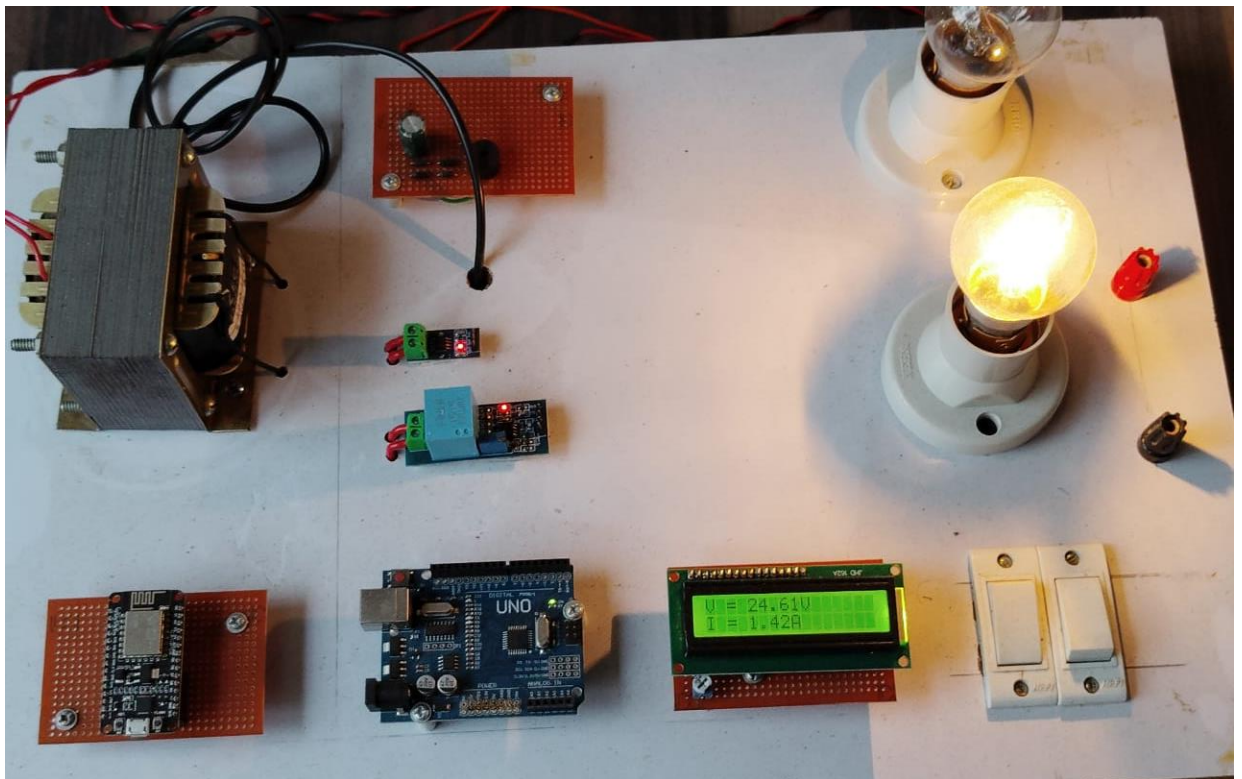
Figure 2: Photograph of the prototype model of transformer health monitoring and theft detection
