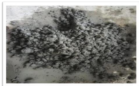
Fig. 3: Mixing of concrete
